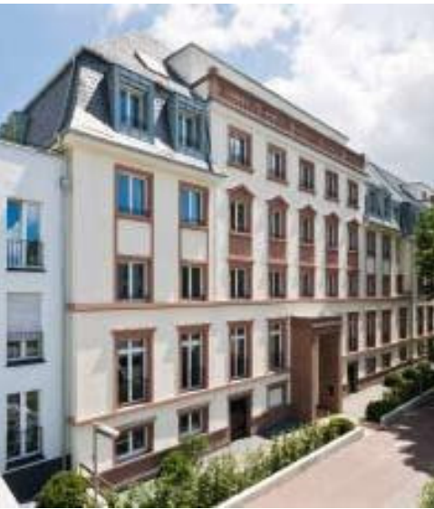
ABG Frankfurt Holding used solid Verofill to create facade details when reconstructing a historical building. Photo: Axel Stephan, Frankfurt a. M., DE
