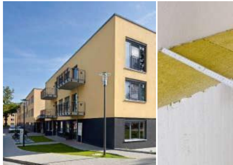
Thanks to StoTherm Classic S1, very dark colour shades are now a viable option. One example is the base level of Hamburg's Asklepios Westklinikum. The system is also suitable for nearly zero-energy and passive houses above the high-rise building limit.
