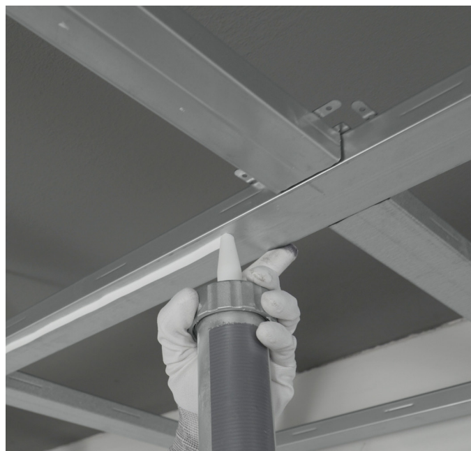
Adhesive application with the adhesive gun
