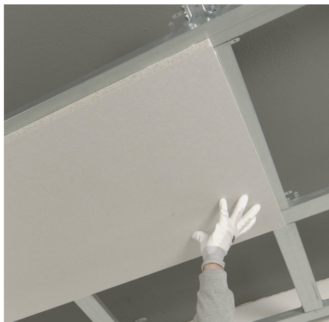
Pressing the acoustic panel into place
