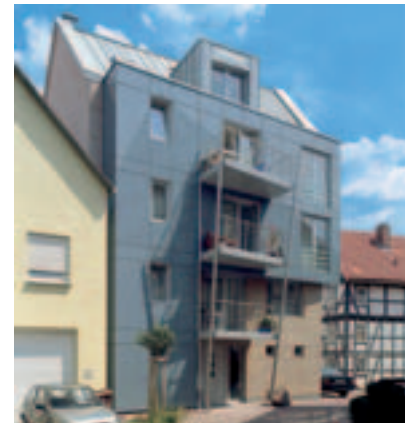
StoVerotec. (Multiple dwelling, D)
