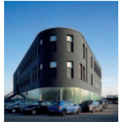
StoVentec. (KLPD police headquarters, NL)
