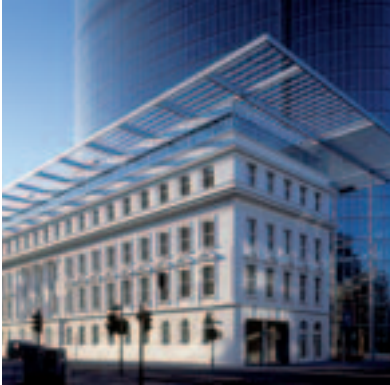
StoDeco Profiles on StoTherm Mineral. (GAP 15 office building, D)
