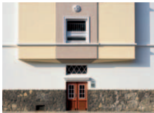
Before and after. (Multiple dwelling, D)
